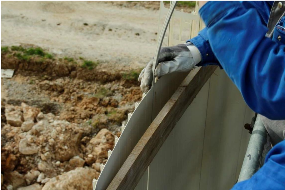
Figure 7. mounting connector for inner panels
