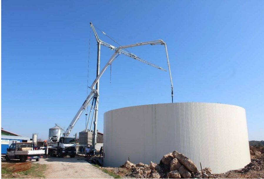
Figure 21. filling the formwork with concrete
