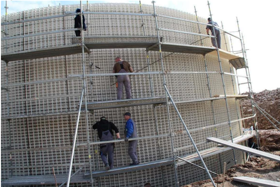
Figure 13. assembly of the vertical reinforcing bars.
