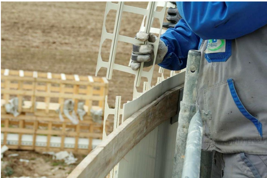
Figure 8. assembly connectors
