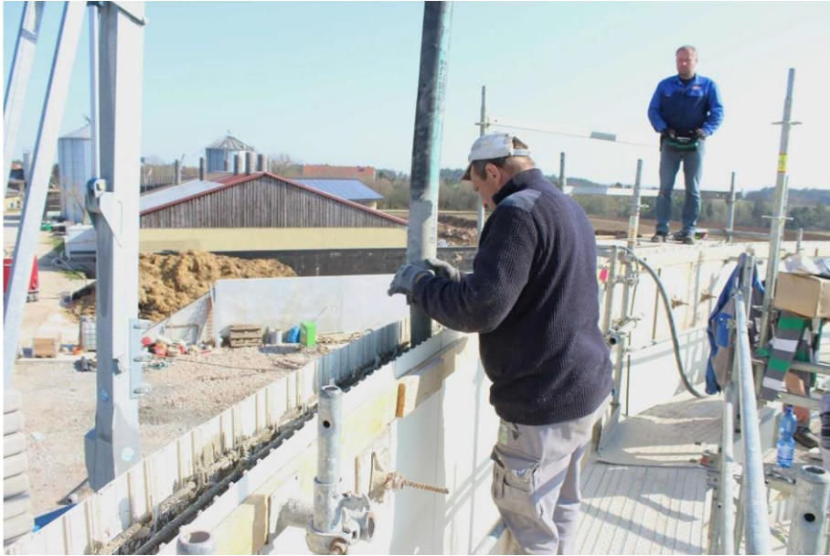
Figure 19. concreting the tank wall
