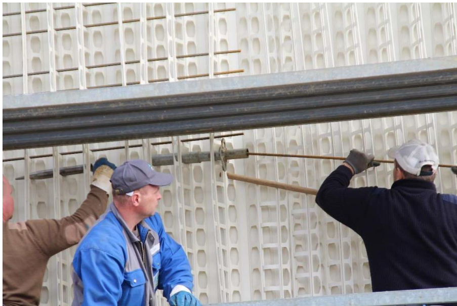
Figure 12. insertion of the horizontal reinforcing bars
