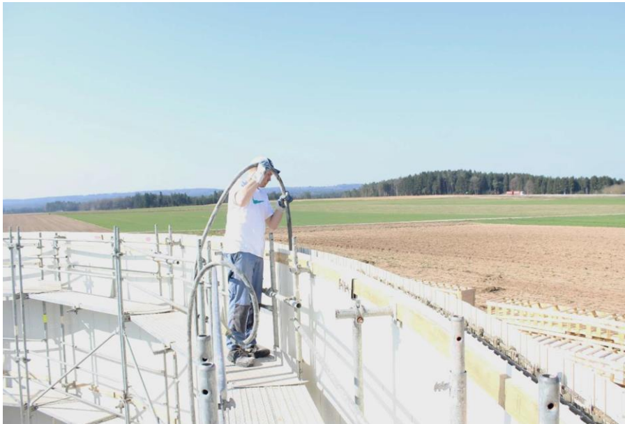
Figure 20. compacting the concrete with vibratory flasks.
