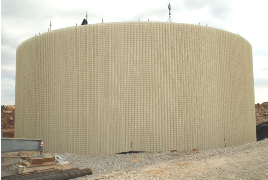
Figure 11. closed inner formwork
