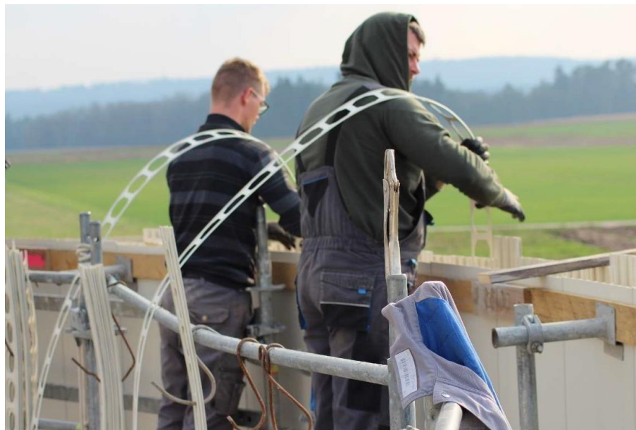
Figure 17. mounting 45° stiffeners on outer panels
