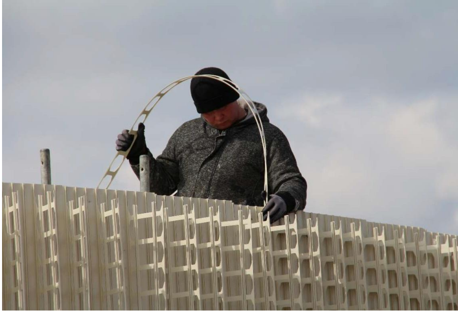
Figure 9. 45° stiffeners assembly
