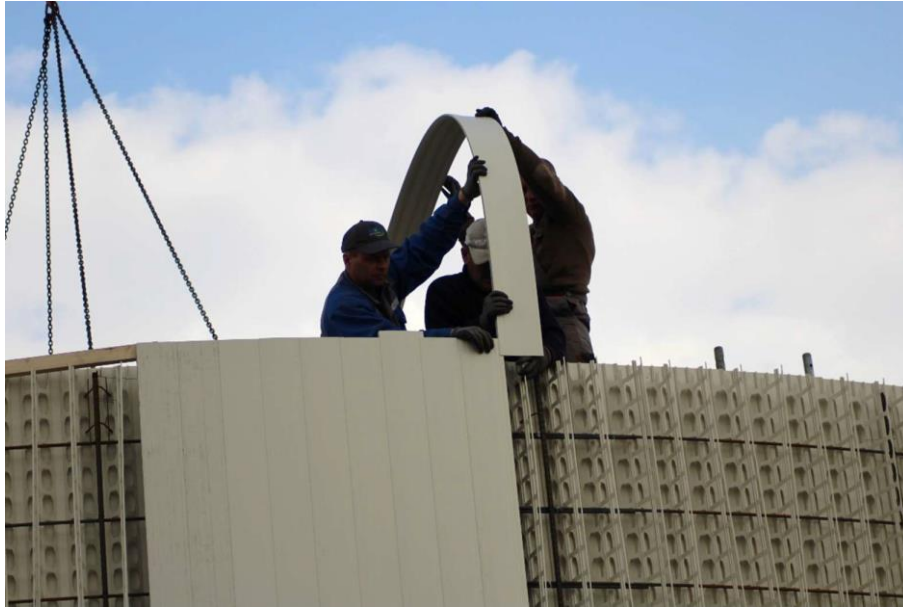
Figure 16. assembly the outer panels
