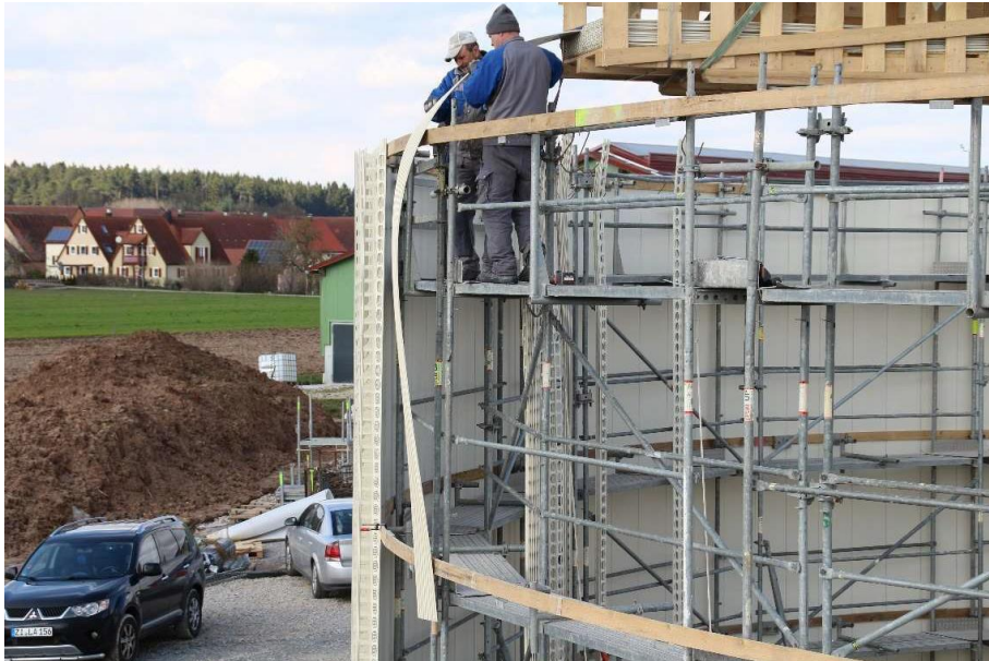
Figure 5. mounting inner panels
